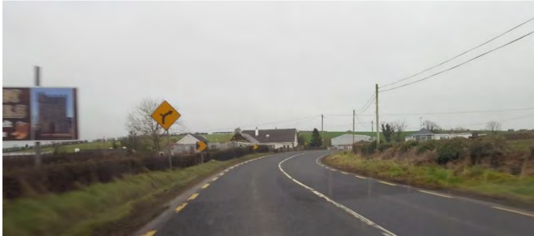
Figure 1-1 Poor alignment on the N14 between Manorcunningham and the R236 junction
